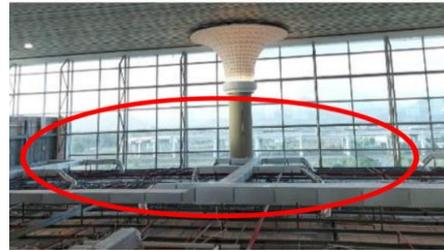
**Gambar 3.** Supply Ducting AHU ke Ruang Concordia Lounge
