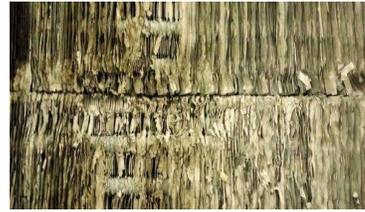
**Gambar 6.** Kondisi Koil AHU 1-1
